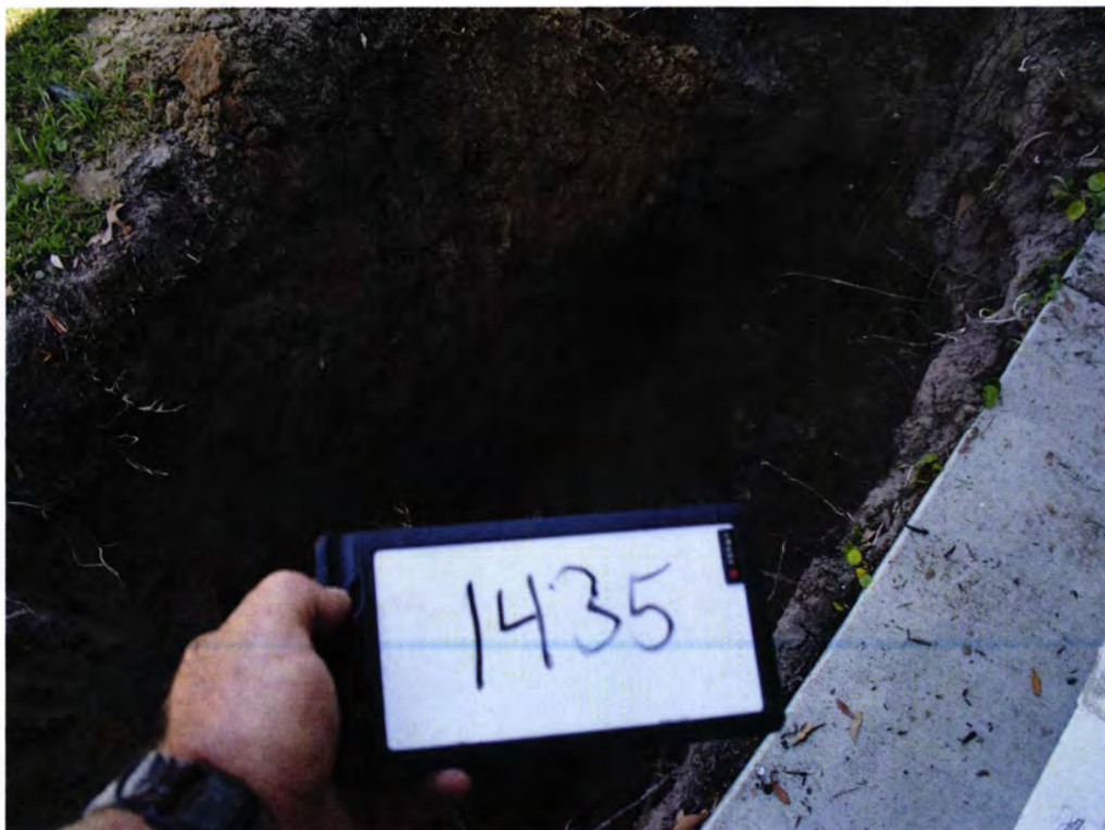
Picture 2: UST 1435Dove excavation pit.
