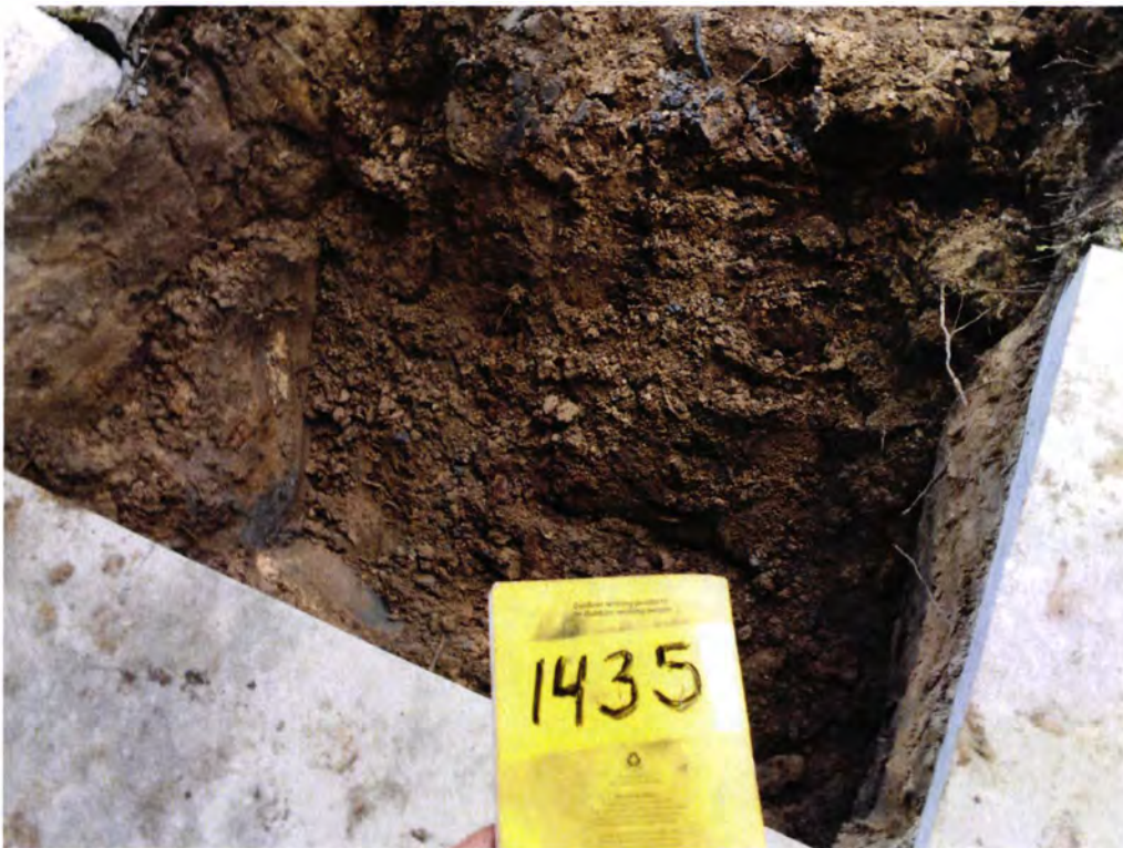
Picture 2: UST 1435-2Dove excavation.
